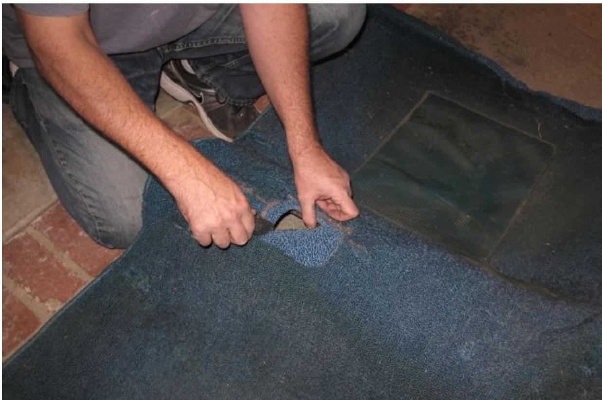
20. Using the old carpet's shifter opening for a template on top of the new carpet, cut the same opening into the new carpet.
