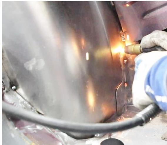
Figure 39 - Tack Weld Flange
