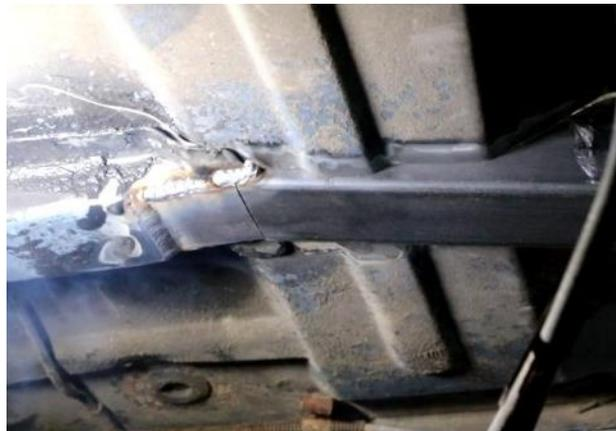
Figure 46 - Weld Sides of Connector
