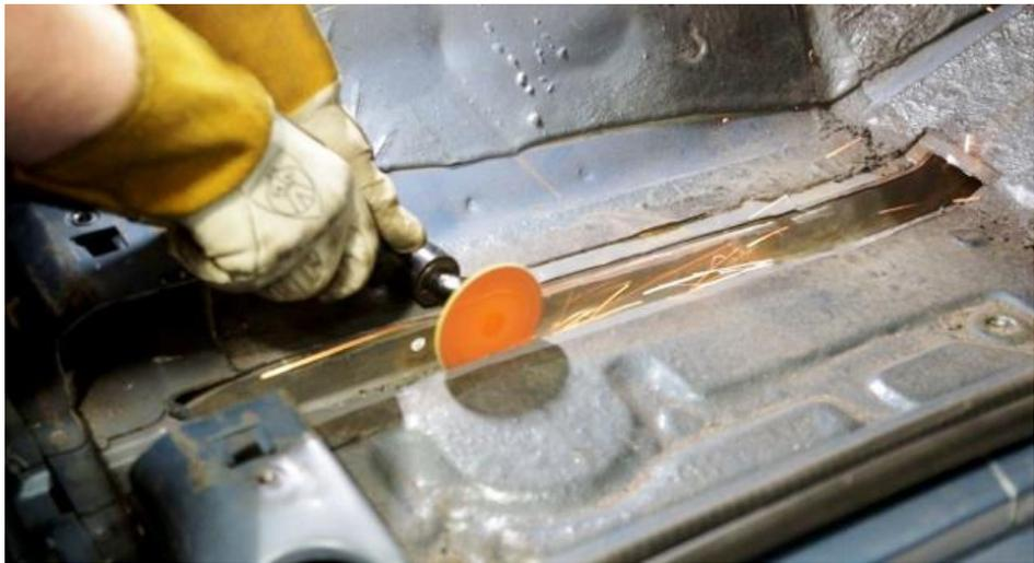
Figure 18 - Grind Cut Lines
