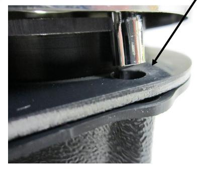
4. Secure the VHX system to the bezel using the four (4) provided 6-20x1" screws in the four bottom mounting holes. Four (4) of the stock mounting screws can be re-used for the rest of the mounting holes.
